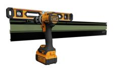
Check level and drive screws at each stud location in both the top and bottom channels.
